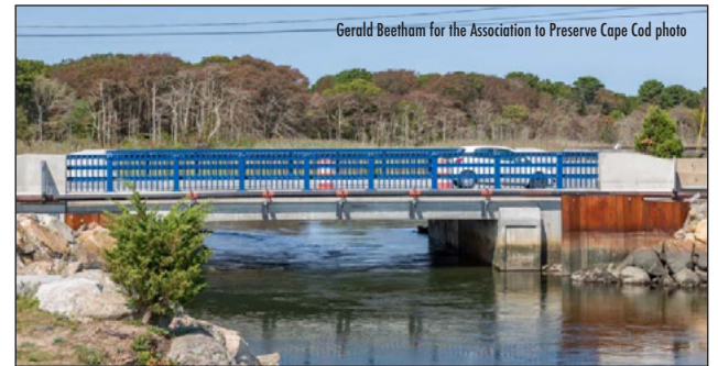
The new 30 foot long bridge crossing the Parkers River at Route 28 in Yarmouth, MA.
